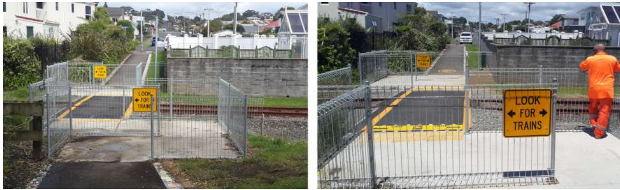
Fig. 1. View of the Cutfield level crossing (Left: Control configuration; Right: Treatment configuration (LEDs) with the protection officer in position for monitoring the rail tracks).
