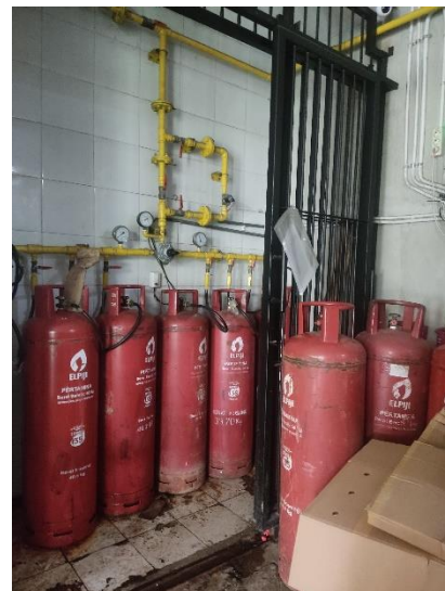
Gambar 18. Area regulator/tabung elpiji area dapur
